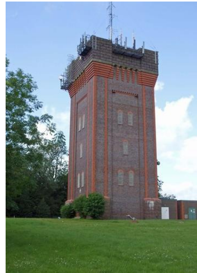
Winhill Water Tower
