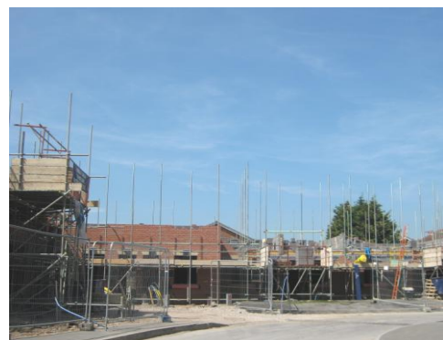
Construction at the old Reynold Chain Site - Horninglow Road, Burton
