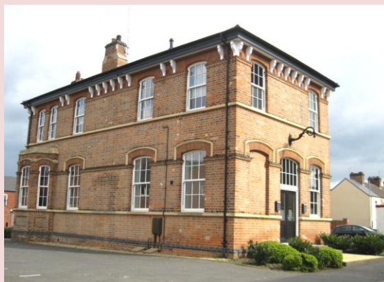
Converted Building within Clarence Street/ Anglesey Road Conservation Area
